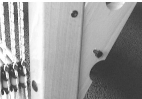
Screw the lag bolt 6 x 30 mm into the pilot hole in the warp beam support, just so far that the thread of the bolt disappears into the wood.
