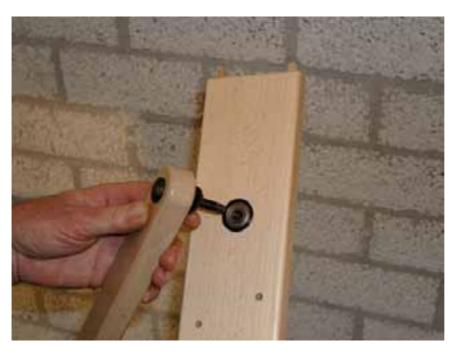
Slide the large washer and then the two small washers over the end of the carriage bolt. Slide the carriage bolt from the outside through the ball bearing in the left side rail. The inside can be recognized as the side with the circular groove for the cloth beam. Put the cap nut on the end of the carriage bolt and tighten with the 13 mm wrench.
