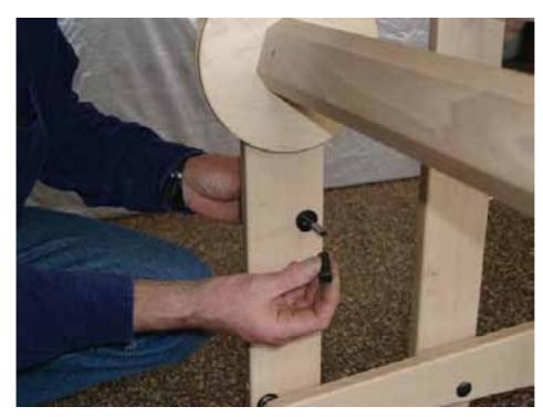
Push the carriage bolt through the hole in the upright of the back part from the outside of the loom. Slide the large washer and the 36 mm spacer bushing over the carriage bolt.
