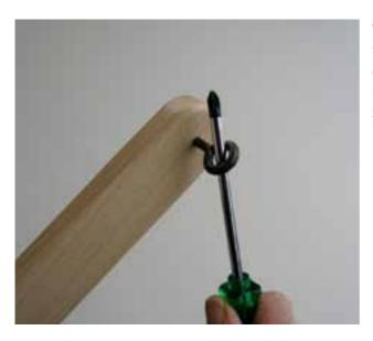
Take the treadle and turn the screw eye in the hole at the end until the threaded part is completely into the wood. The picture shows how the eye needs to be located relative to the treadle.
