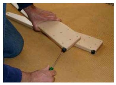
Take the two treadle sides from box B. Attach the buffers with the 4 x 21 mm screws onto the angled corners.
